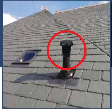
Poly-Air installed on a roof ventilation pipe.
